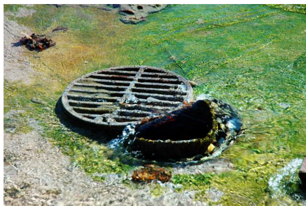
The compound has diverse applications - surface coating would reduce severe industrial fouling and corrosion.
